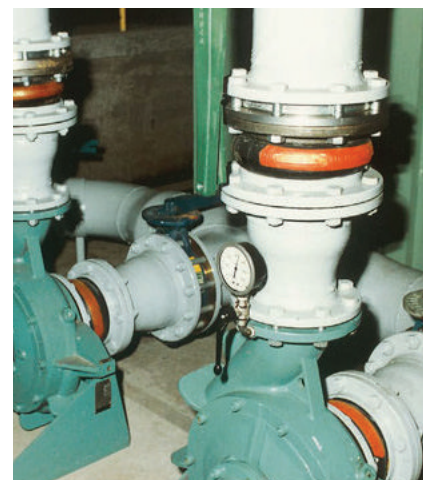
STENFLEX® type A-1 used at pumps
