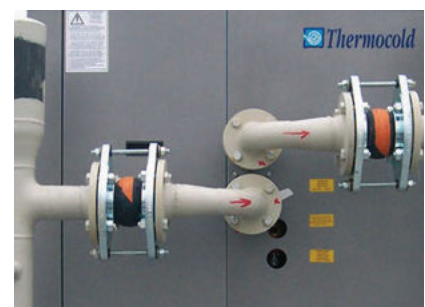
STENFLEX® type AS-2 at an industrial plant
