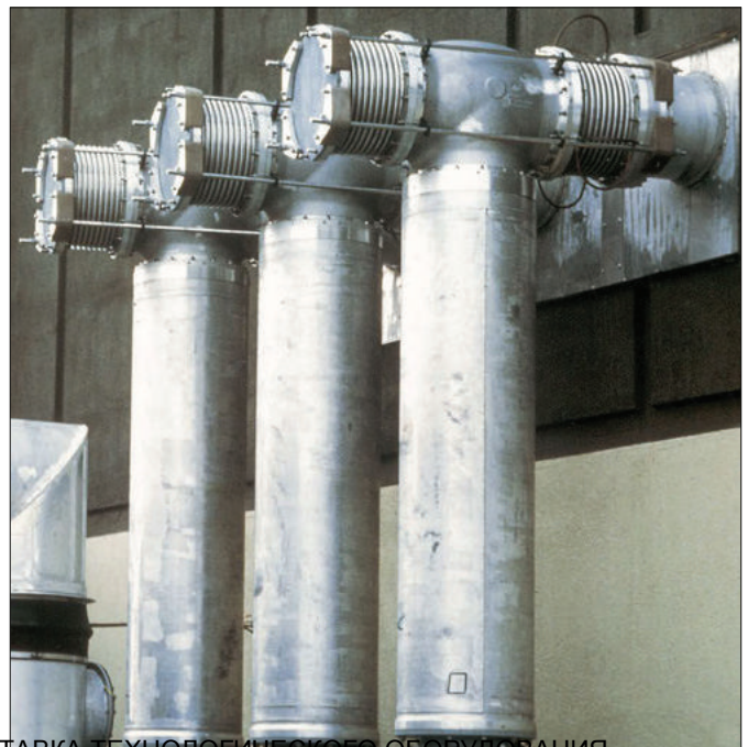
Restrained STENFLEX® stainless steel expansion joints type SF-25 to absorb
