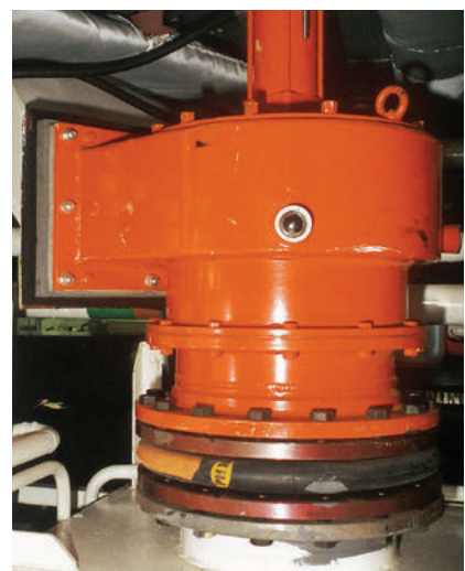
STENFLEX® type B-1 for compensating large movements
