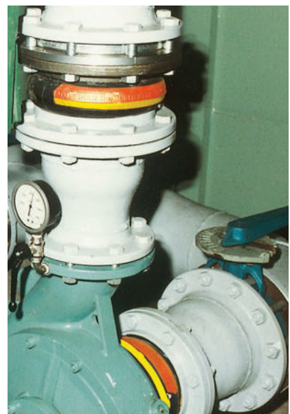
STENFLEX® type AR-1 used at pumps
